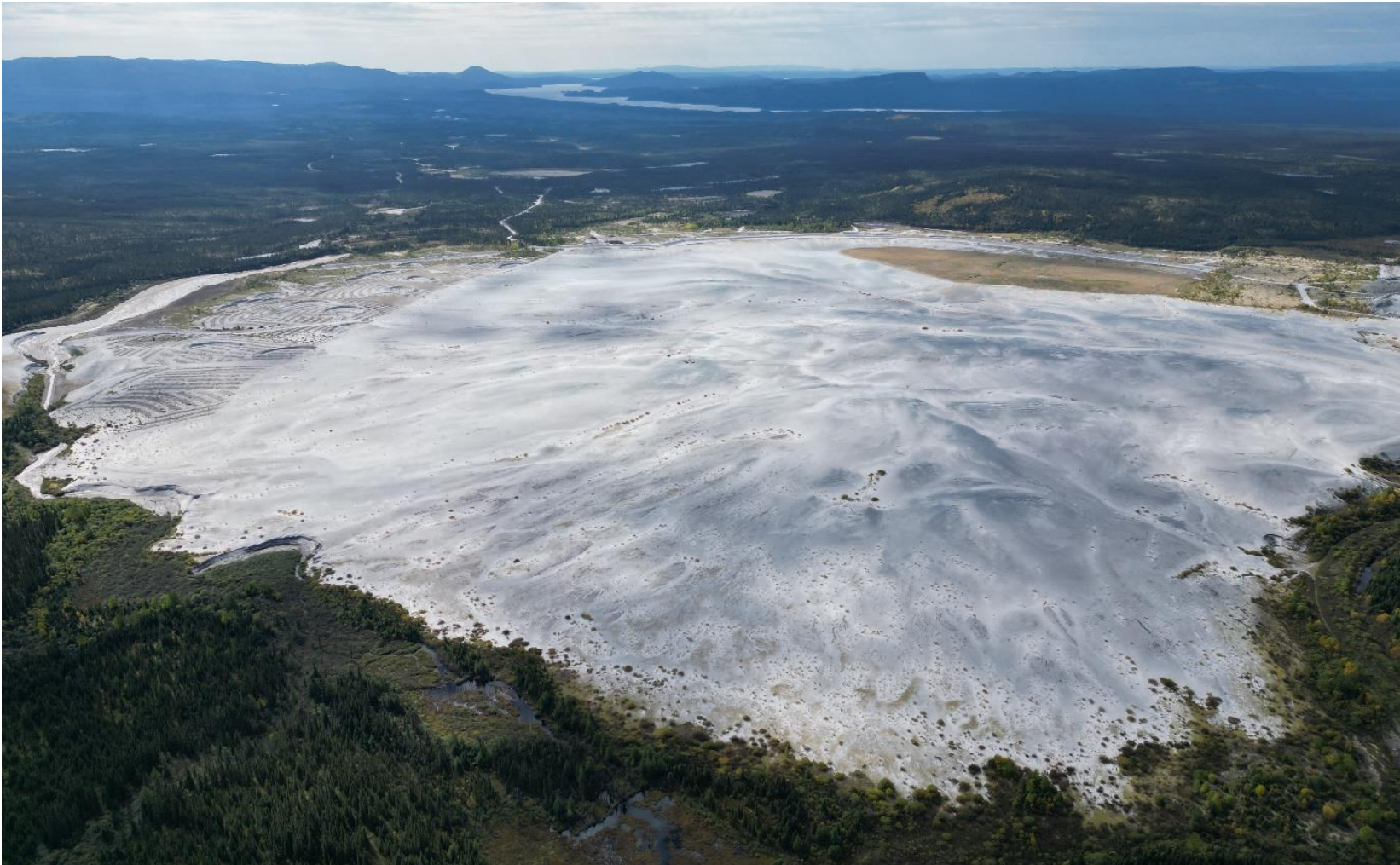
Figure 5.5: Larger Project area view looking southwest (source: Sonic Edge drilling company drone, 2023).
