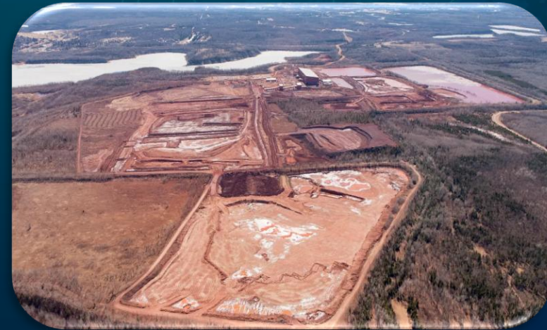
Plant 4 Overhead Photo
